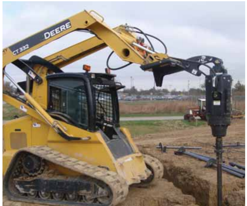
Long reach skid mount used to install helical anchors.
